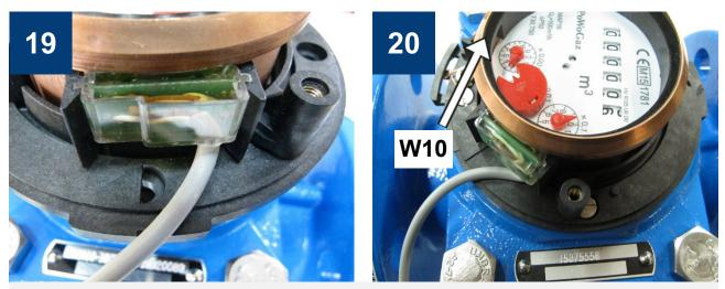
View of the NK transmitter installed in the position to transmit the pulses from the magnet fixture installed at the x 0.01 indicator position (DN50-125): pulse rate at 100 L = 1 pulse. If the magnet fixture is located at the x 0.1 indicator position (DN150-250) or the x 0.1 indicator position (DN300 twin indicator front plate), the pulse rate is 1000 L = 1 pulse.
